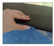
Angle and tuck gasket into channel in edge of counter top.Insert graphic gasket all the way around.
